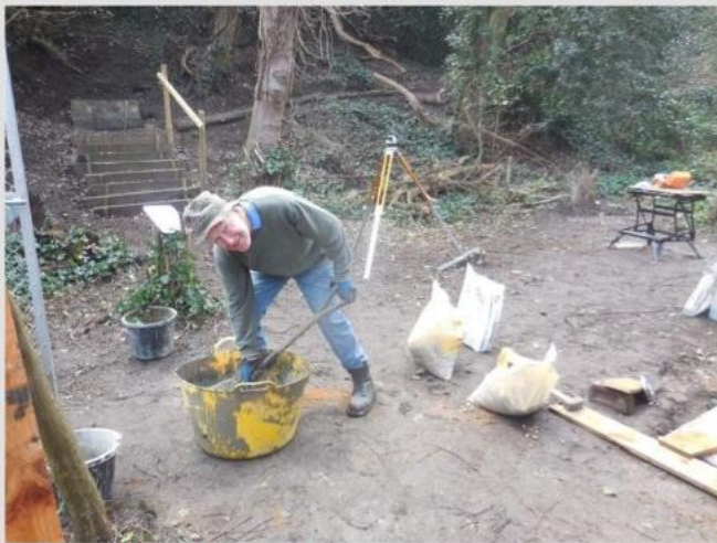
Frank laying a foundation. Picture, Andrew Slade
